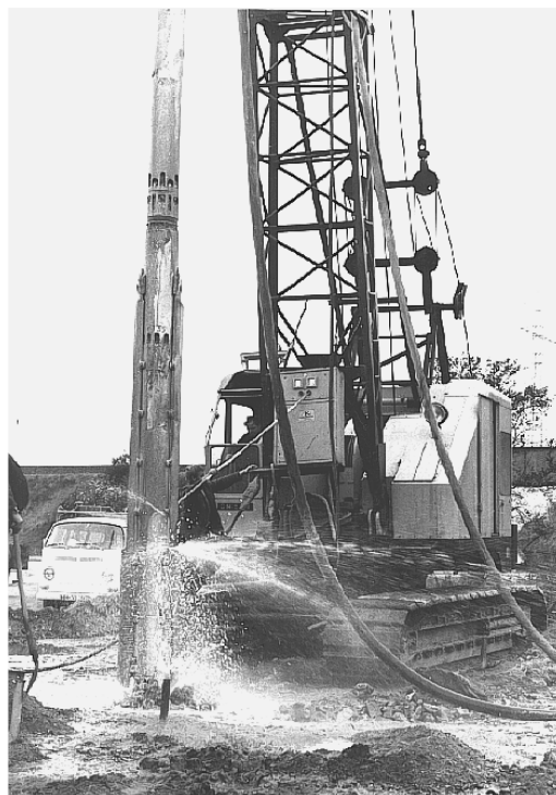
Figure (1): Dynamic compaction using a vibrating probe.
