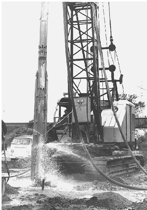
FIGURE (1): DYNAMIC COMPACTION USING A VIBRATING PROBE.
